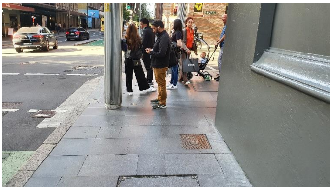
Figure 23: Kent / King St intersection – south-east corner, showing pinch point of the lamp/traffic signal pole.
